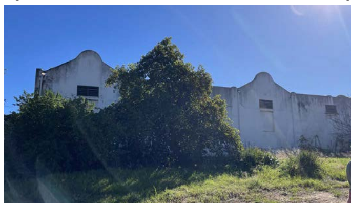
Fig 23C: Northern elevation of the northernmost barn building.
