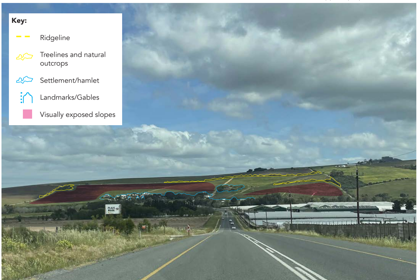
Figure B: View from the Annandale Road, above the strawberry farm, towards Lynedoch. White dotted line indicates approx. property boundary. This view indicates the high visual exposure of the upper slopes and east and west "flanks" at Lynedoch.
