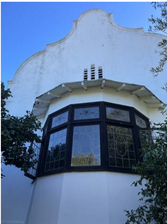
Fig 23H: Detail of a projecting lead-glass bay window.
