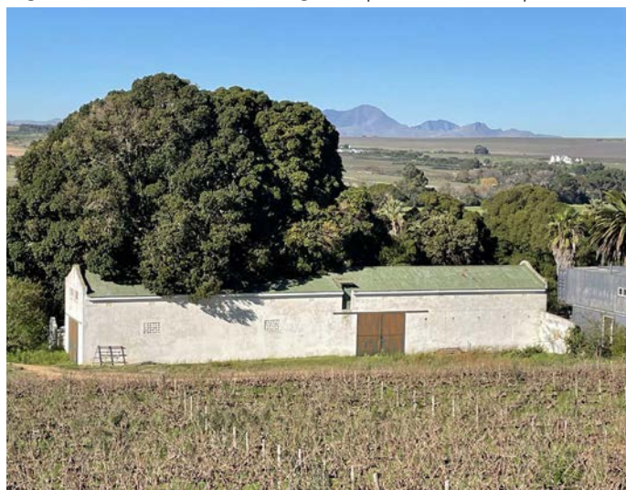
Fig 23B: Southern elevation of the southern-most barn building
