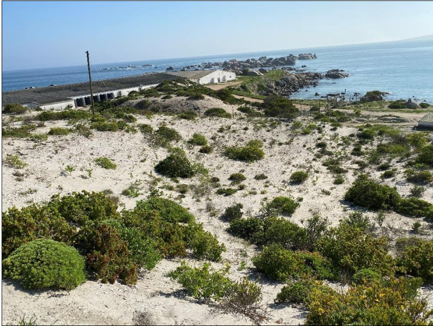
Figure 21. Site 035. View facing north west with the crayfish factory in the distance. Note the Eskom line which cuts across the dune basin
